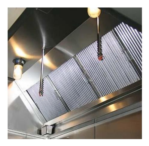
FILTERS ARE TESTED TO THE ASTM F2519-05 GREASE PARTICLE CAPTURE EFFICIENCY OF COMMERCIAL KITCHEN FILTERS AND EXTRACTORS.
